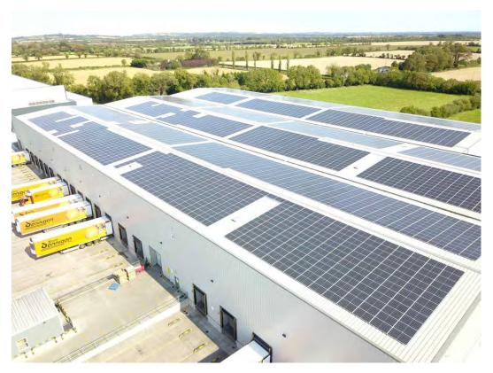
Figure 2-4:Example of roof mounted panels from another site (Dennigan site)
